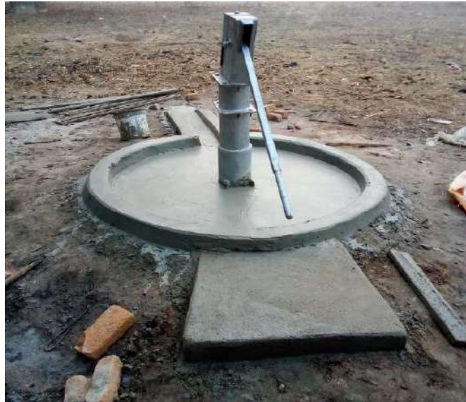
3 Nos of Handpump installed in PH villages.
